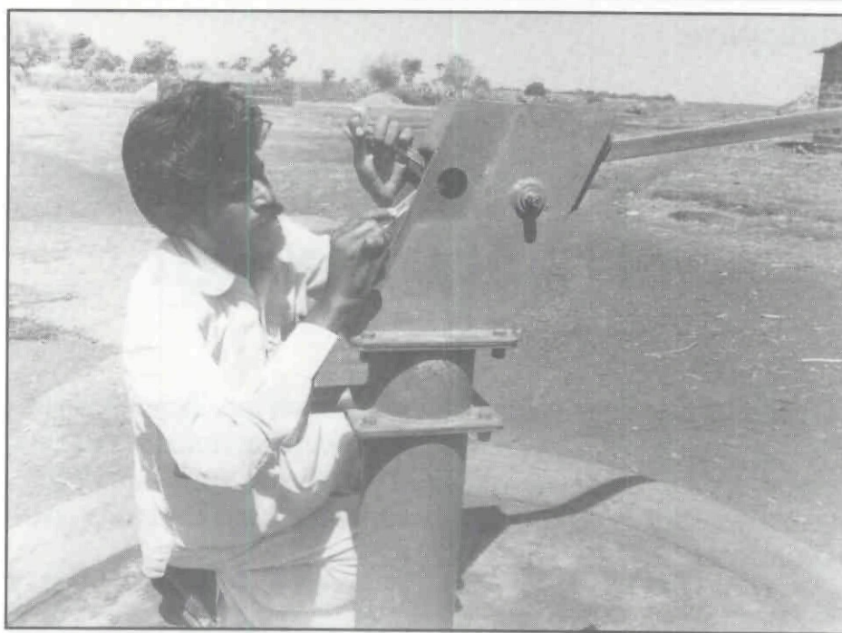
"Every week, Sri Laxman uses the spanners given him after his caretaker's training to tighten the nuts on the Bilalpur handpump." ICF 9299/Nagarajan
