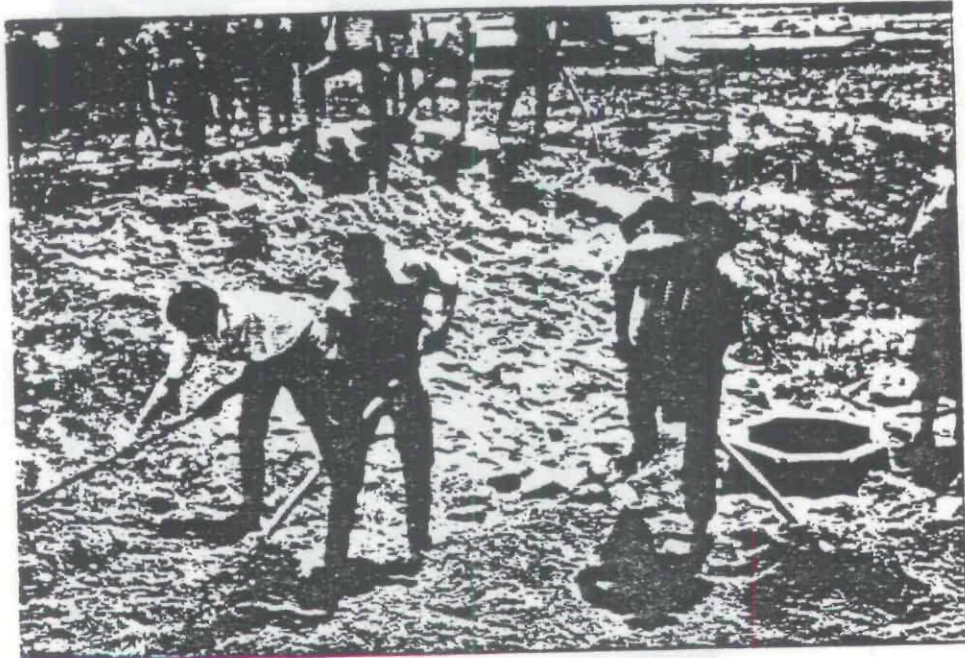
Filling in with dirt
