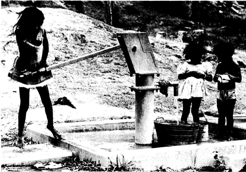
A simple, dependable and maintainable water hand pump known as the India Mark II has been developed. These pumps have brought water supplies to thousands of previously-deprived communities. (Unicef/Holbrooke)
